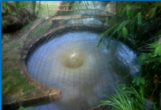
↑ The vortex energy plant supplying electricity for the Green School, Bali. www.greenschool.org
