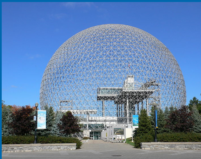
The Geodesic Dome at the 1967 Montreal International Expo. Interspersed among the hexagons are some pentagons to allow for curvature. 5 + 6 = spherical geometry.
